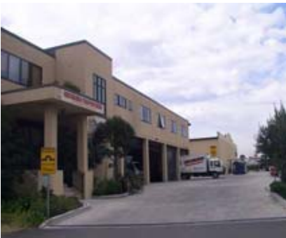
Surveillance must be provided to vehicle routes, as in the above industrial building.
