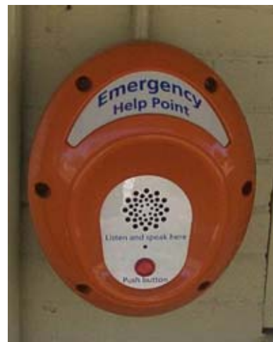
Emergency help points in larger developments can assist in addressing immediate safety risks as well as acting as a deterrent to other undesirable activities such as vandalism (which may be reported by observers).
