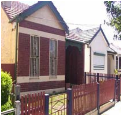
Security measures such as grilles should not preclude fire safety (House 1) or obstruct surveillance from the dwelling to the street (House 2).
