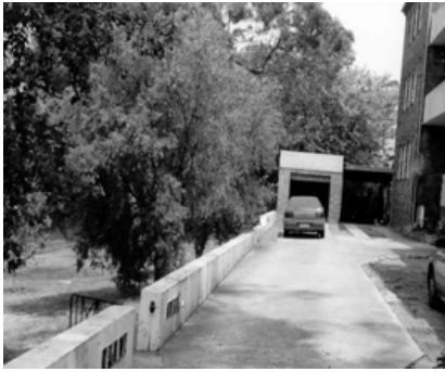
Public and private areas must be clearly delineated as in the case of this public park and adjoining residential development.
